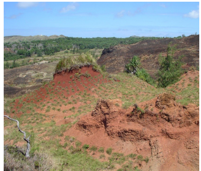
Fig. 6 This photo shows grass plantings on a military land restoration project. Grass will offer greater protection from erosion than will trees in these soils. Note the soil remnant indicating that at least about 2 meters (6 feet) of soil has been removed from this landscape. Also note the recent burned area in the midground of the photo. Credit: Bob Gavenda
