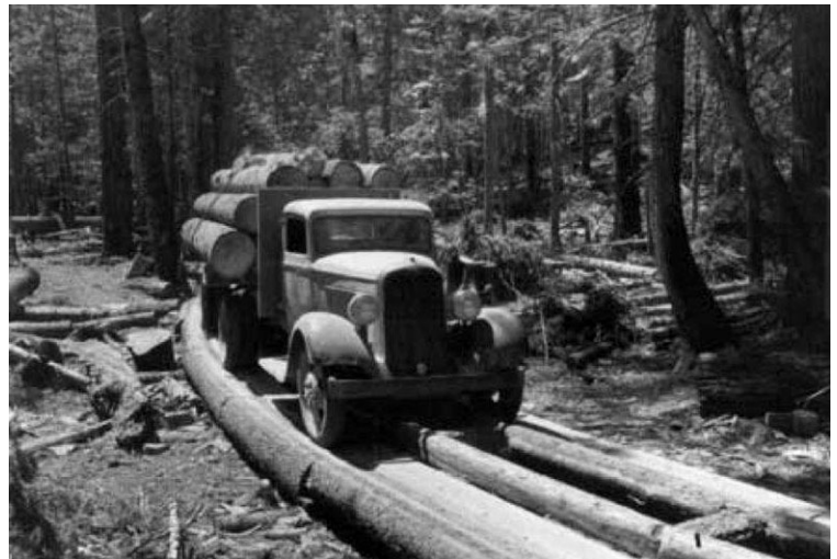
Fig. 4. Some of the best timber in northern Idaho is produced on Threebear Soil. This USDA-Forest Service photo from 1935 shows a loaded logging truck in the Clearwater National Forest where Threebear soil occurs. Credit: USDA Forest Service: http://foresthistor.org/ASPNET/Publications/first_century/sec6.htm .
