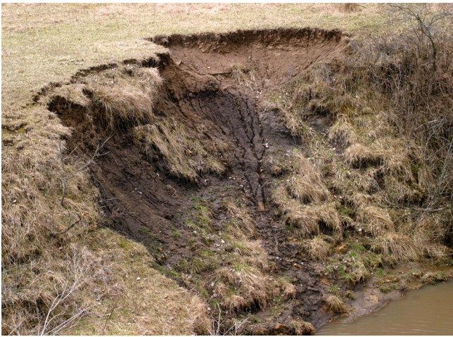
Figure 4 Example of erosion. Credit: Adobe Stock.
